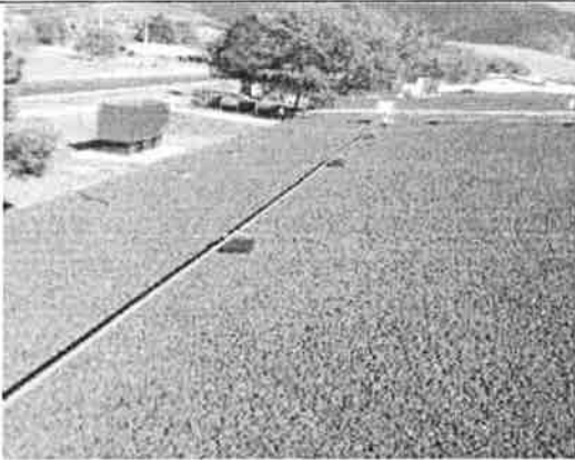
Overview of the roof
